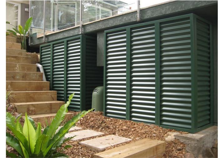
Figure 133: Concealed tanks integrated with the design.
