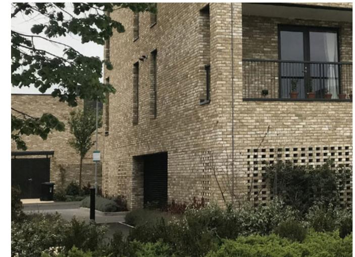
Figure 75: Undercroft parking combined with planing and feature brickwork at ground floor level.
